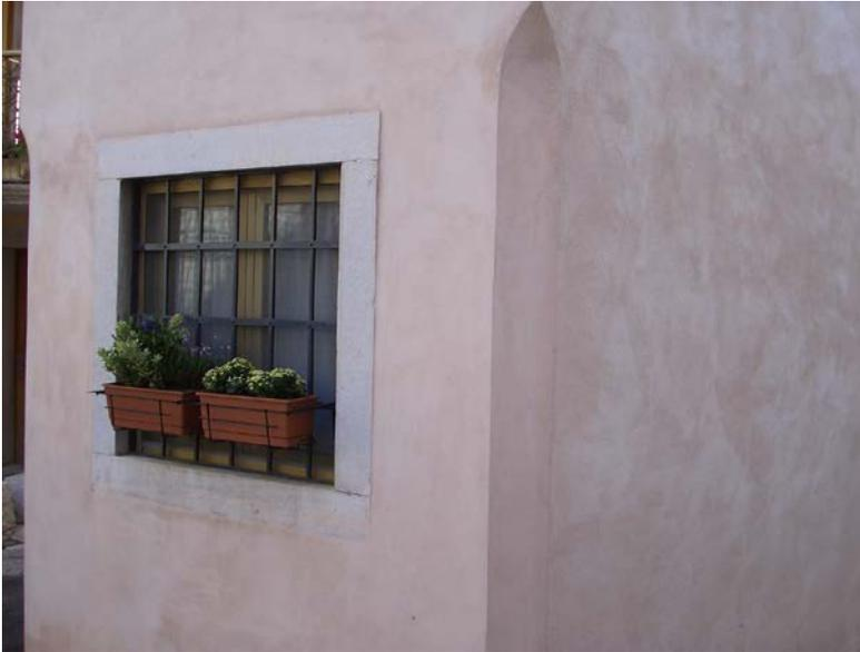
Malta Grezza & Malta Fine produce this characteristic pink tone when *Cocciopesto* is used to provide added water-resistance and faster set.
