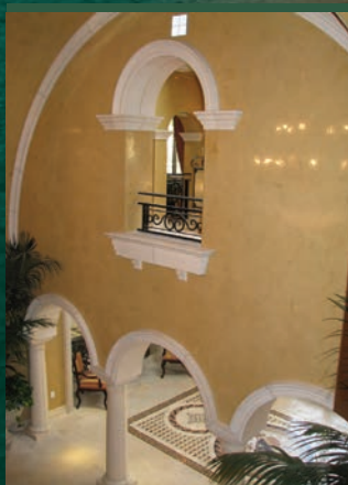
Solution Old Mission Plastering: Orsini Apartments, Los Angeles, CA
